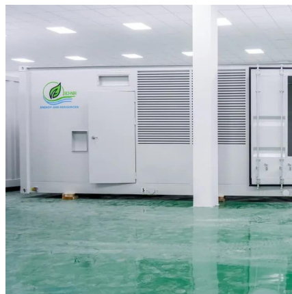
Energy storage container, BESS container
