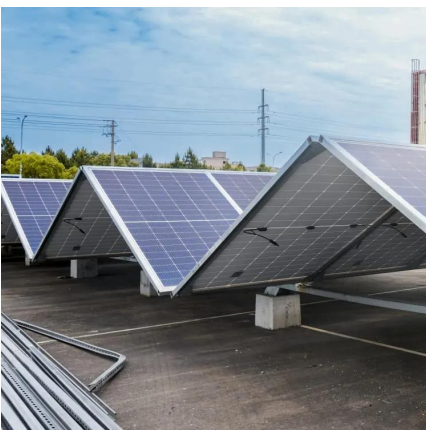
Pyongyang power plant energy storage station
