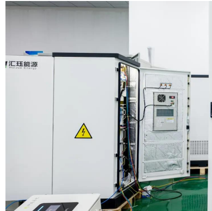
100KW Energy Storage Container
