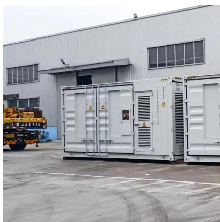
**Hybrid Container Solar Battery Energy Storage System
