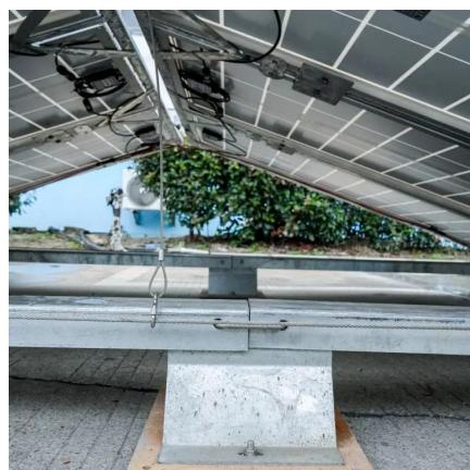
**Film-type Perovskite Solar Cells Installed in Umekita**
