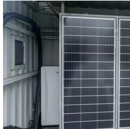
Indoor Wall-Mounted Energy Storage Battery
