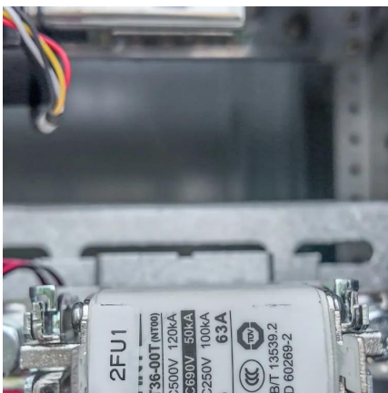
2kWh Vestwoods Power Station in Kenya
