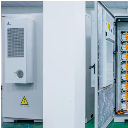
Ghana photovoltaic module combiner box
