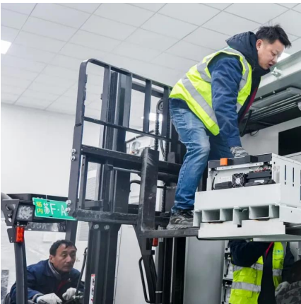
30kW Solar Hybrid System for Egyptian ...
