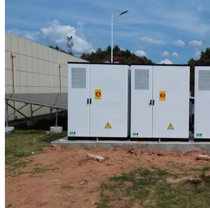
30kW Solar Water Pump Inverter in Fayum, Egypt
