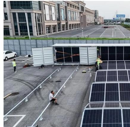
[100kW Dual Axis-solar Radiation Tracking \(DART\) Solar Farm](#)
