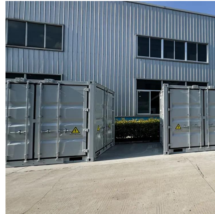
Photovoltaic energy storage charging pile
