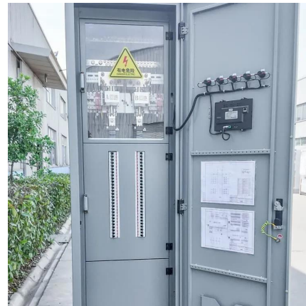
LLVD & BLVD in Base Station Power Cabinets
