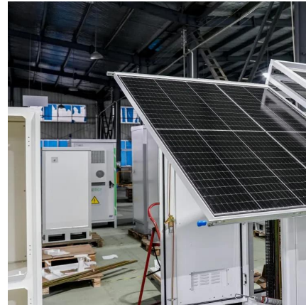
Portable Off Grid 500kwh Energy Storage ...
