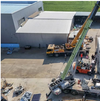
Containerized Energy Storage System BESS ...
