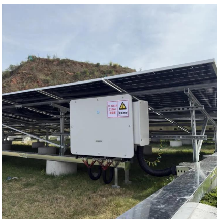
solar battery storage
